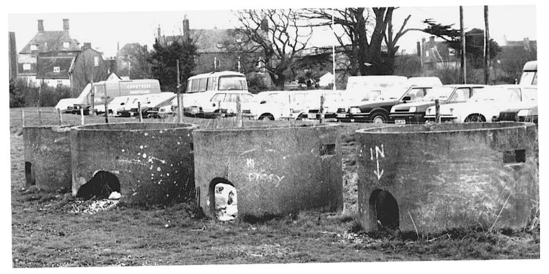
Four circular 'NORCON' concrete firing positions, 7ft diameter and 4.5 ft high were built by the East Street viaduct and on the railway embankment by the River Stour to defend the town from invasion from the East.
