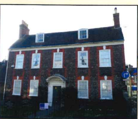
Lime Tree House in The Plocks has fine purple brick work with red dressings. The Plocks was a holding area for sheep on their way to Sheep Market Hill.
