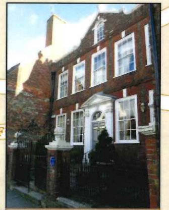
Eastway House built for John Ayliffe, a merchant, is notable for its five bay brick façade, and various decorations of urns and balls, being set back from the street behind railings.
